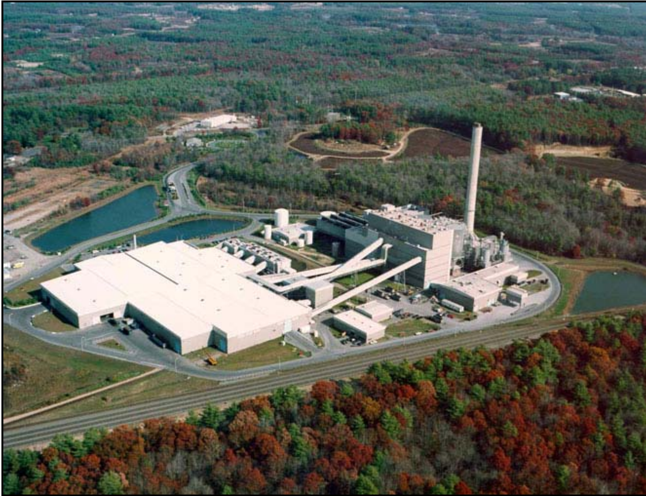
SEMASS Resource Recovery Facility Rochester, Massachusetts Developed by Energy Answers
