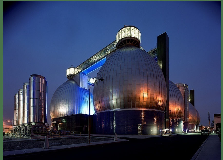
Newtown Creek Digesters – New York City
